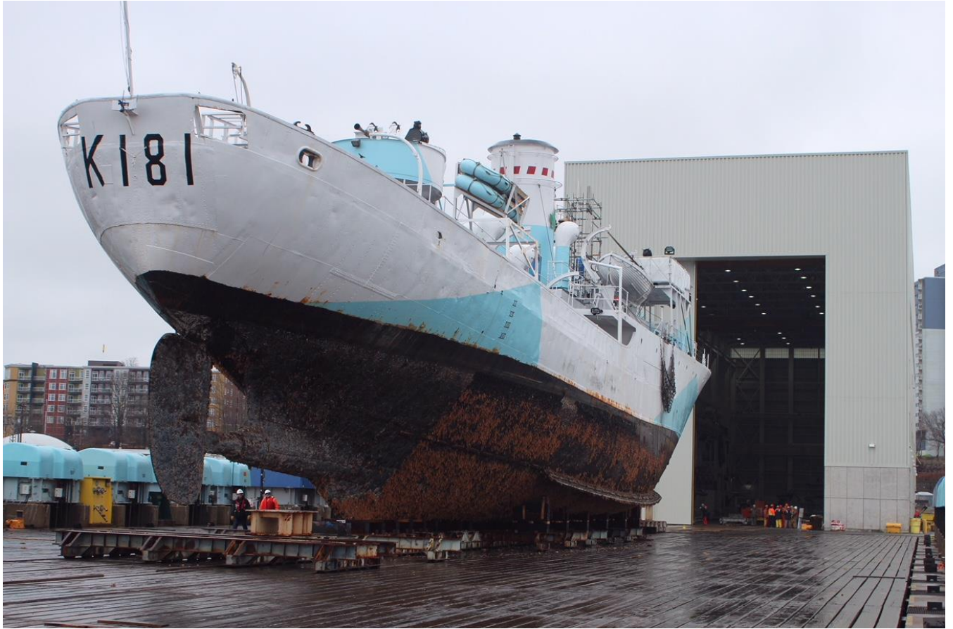
HMCS Sackville undergoes hull cladding in submarine shed 2021.
