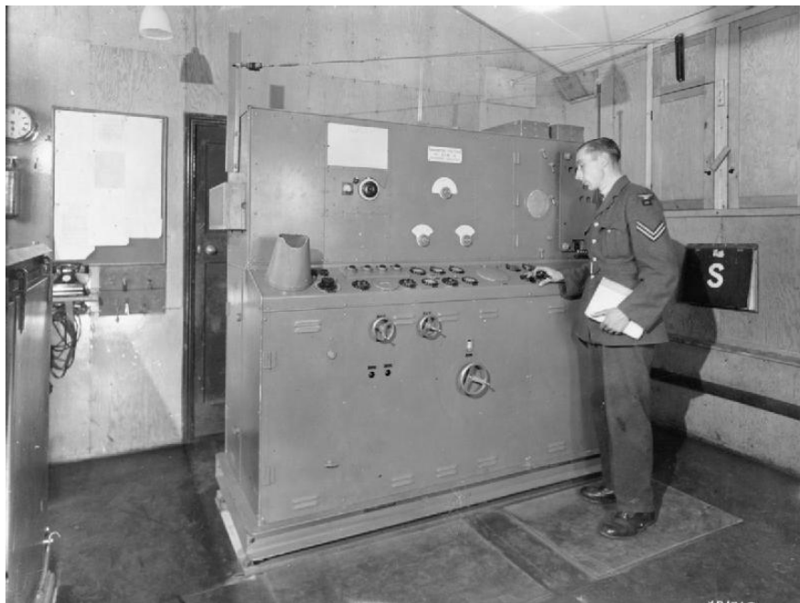
Metrovick Radar Type T3026 transmitter assembly
